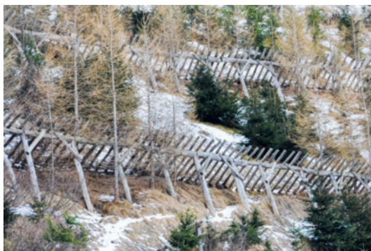
Figure 51 SLF-type wooden snow rake combined with afforestation to protect a transport route.
