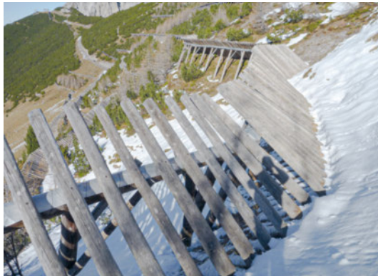
Figure 47 (right) Tripods on a slope prone to gliding snow in a settlement area.
