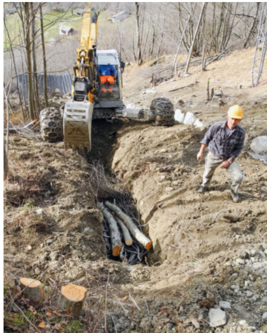
Figure 14 (left) Drainage construction using deadwood fascines.
