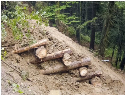
Figure 71 (left) Full coverage can greatly extend service life even if less durable timber species, such as spruce, are used.
