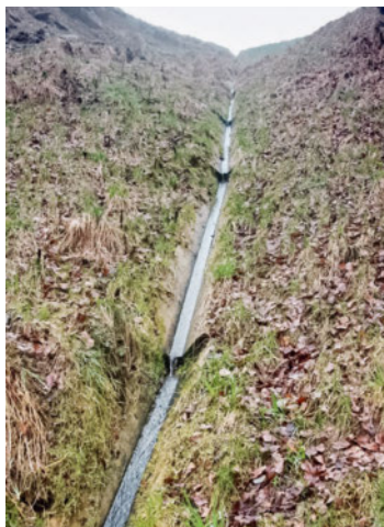
Figure 12 (left and centre) Examples of the construction of a V-channel.
