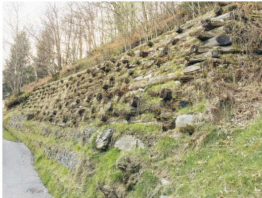
Figure 30 (right) Decayed and compressed cross-sections of the wooden crib's transverse logs.
