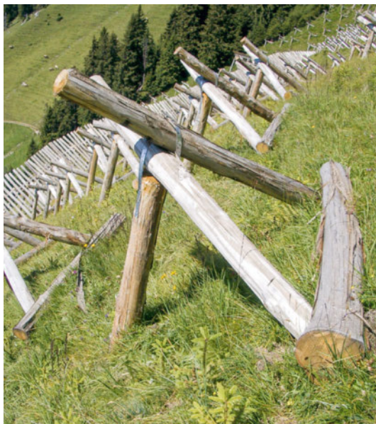
Figure 55 Tripods with upslope sill protect young stands against gliding and creeping snow.
