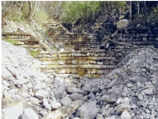
Figure 40 Infill with stones: Wooden check dam after exposure to debris flows.
