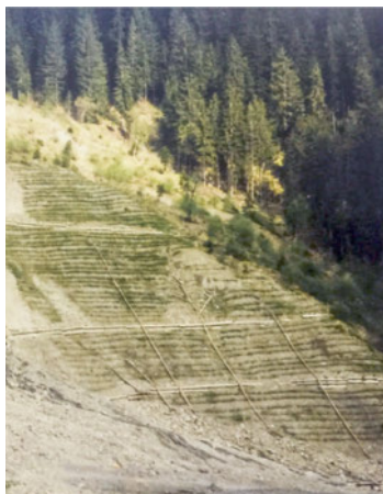
Figure 31 Vegetation development over time on a slope covered with wooden control structures in Arieschbach, Grisons, Switzerland. Left: 1998, Centre: 2005, Right: 2017.
