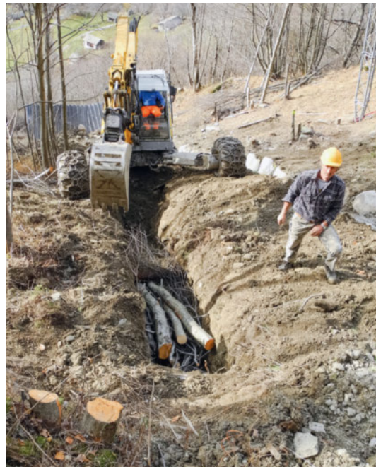
Figure 14 (left) Drainage construction using deadwood fascines.
