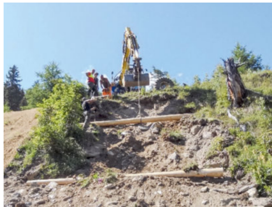
Figure 19 (left) Construction of rear- anchored wooden logs to stabilise an embankment.
