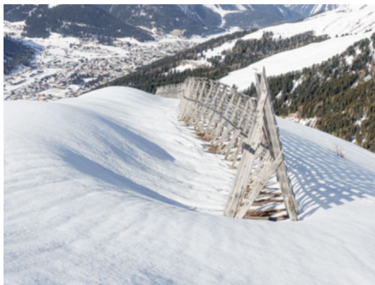
Figure 59 Snowdrift fence made of timber elements. A large snow deposit has formed in the lee of the fence (to the left in the photo).
