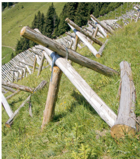
Figure 55 Tripods with upslope sill protect young stands against gliding and creeping snow.
