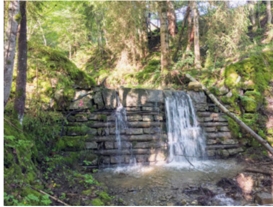
Figure 67 Check dam in the Schaferabach stream in the municipality of Plaffeien, Switzerland. Some of the dams in the Schaferabach are known to have been built between 1940 and 1945. This means they have served unaltered for more than 75 years.
