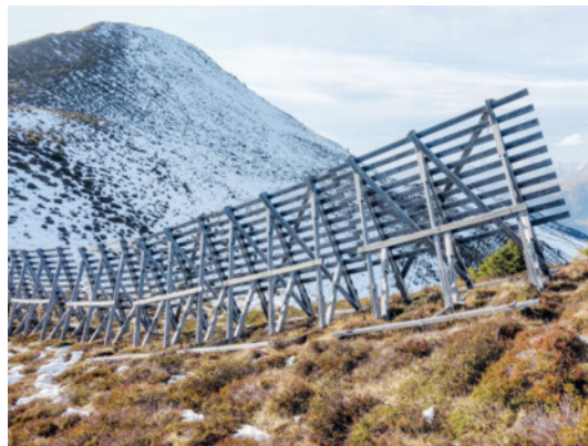
Figure 48 (left) Snowdrift fence made of 5 m long timber elements.
