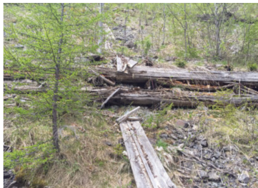
Figure 9 (left) Terrace made of now decomposed single-walled wooden cribs combined with a water drainage channel in Arieschbach, Grisons, Switzerland.
