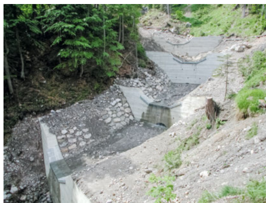
Figure 61 (left) Concrete check dams on the Mauerbodenbach constructed in 2006/2007 [65].
