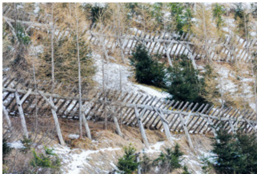
Figure 51 SLF-type wooden snow rake combined with afforestation to protect a transport route.
