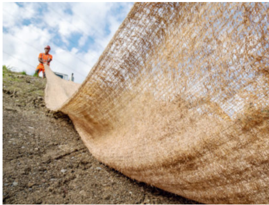
Figure 8 Erosion protection with slope erosion control matting made of wood wool.
